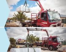
Roofing being positioned on the driveway (roofing pack is approximately 2.5m in length).
